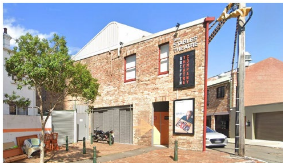
Photograph 2: Northern facade of the existing Stables Theatre, looking south (Source: TZG Architects)
